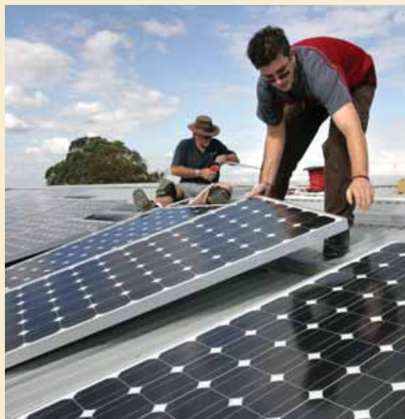
Installation of solar panels at Tirimoana Primary School
