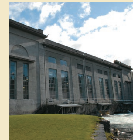
Tuai Power Station Part of the Waikaremoana Power Scheme
