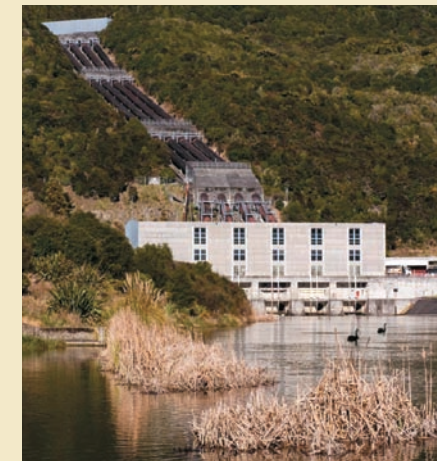
Tokaanu Power Station Part of the Tongariro Power Scheme
